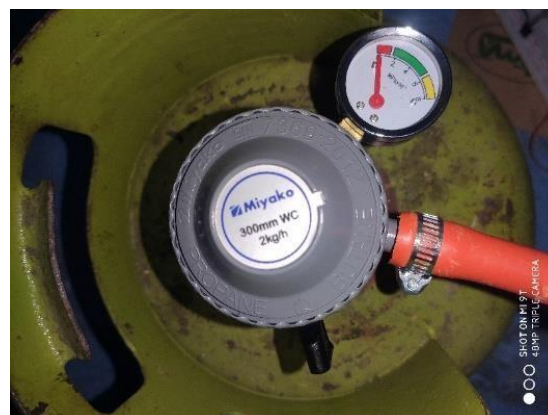
Figure 8. Second regulator with valve conditions not yet locked
